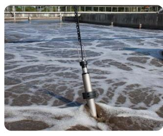
(Sensor holder EH/U 170 in combination with swing mounting assembly EH/F 170-1,5)
